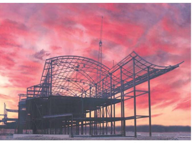
**Both pages:** Steel joist design possibilities are endless when you consider various joist profiles, loadings and applications. These possibilities rise from four distinct joist profiles: gable, bowstring, scissor, and arch. An architect's vision often can be cost-effectively met during the early design stage of a project, based on one of these four types, a variation of one type, or a combination of types.
